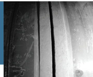
1230 kg Sikadur 30, 20 kg Sikafloor 156 (Primer) and 20 kg Sikagard 63N (Coating) were used to build up the pipe ends.
