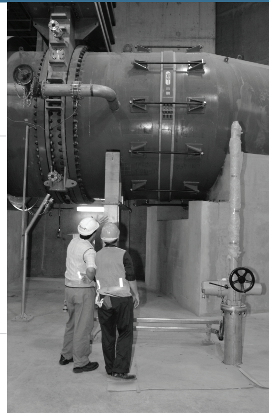
Four 3.6 m diameter couplings were installed.
