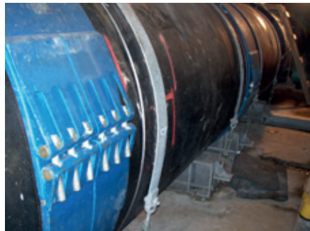
A two-piece housing was used, allowing a subsequent installation without moving the pipes
