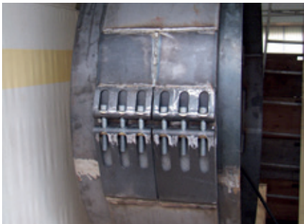
The STRAUB-OPEN-FLEX 4H 1670 mm used for installation and pressure test
