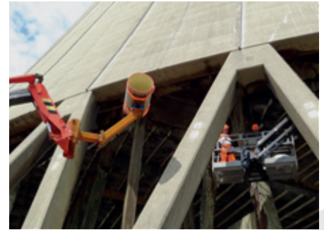
Preparing a piece of pipe for installation
