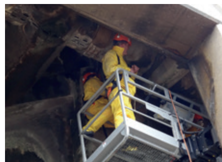
Difficult installation conditions due to the 13 m height and confined space
