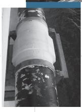
Finally, wax tape corrosion protection was applied to the coupling and the pipe.
