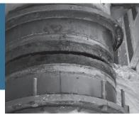
When being exchanged, the old couplings were cut open lengthwise on both sides and the resulting half shells were then removed.
